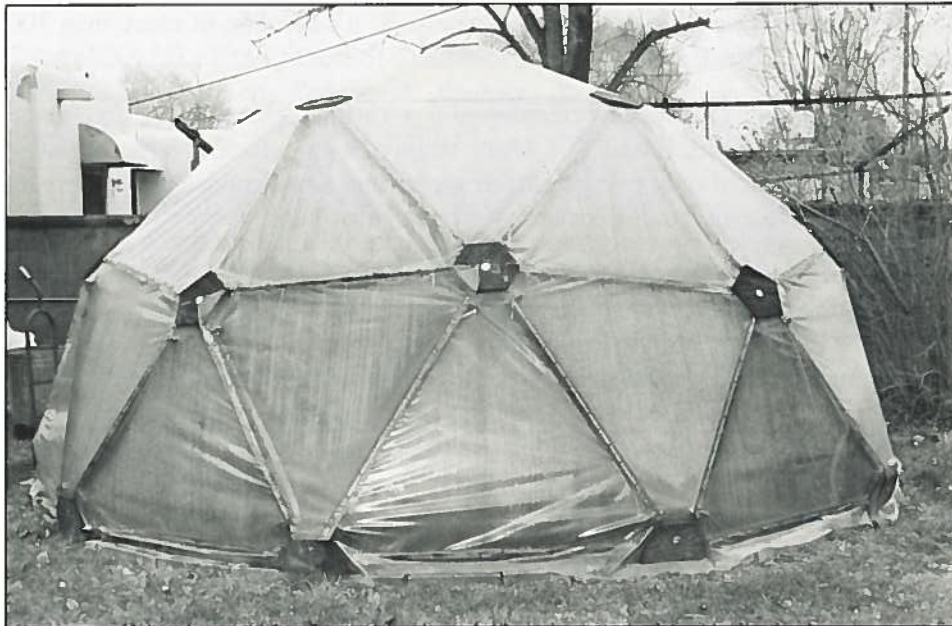
Fig. 7. My greenhouse from the south. Compare with model in figure 6. Struts are joined at hexagonal or pentagonal hubs, pre-drilled using a template and bolted through. The dome rests on a ground-level cinderblock foundation, but can be lifted off. It has withstood 80-m.p.h. winds.
